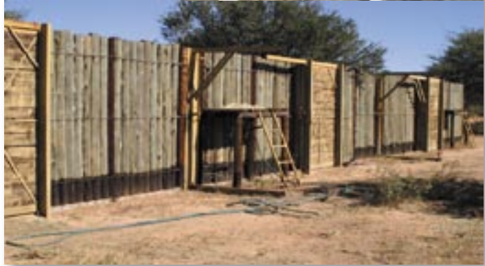
(Top) Round bar bent to prevent rhino from injuring itself. (Bottom) Cable bomas are not recommended. The viewing platform is helpful to observe and feed the rhino.
