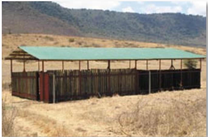
Note slope of land and high, slanted zinc roof for good shade, protection and ventilation.
